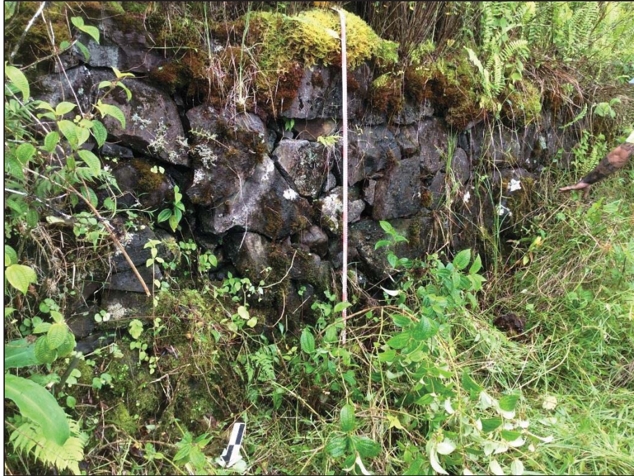
Figure 54. Oblique profile view of a stacked basalt stone wall at the Banana sluice gate, view to south
