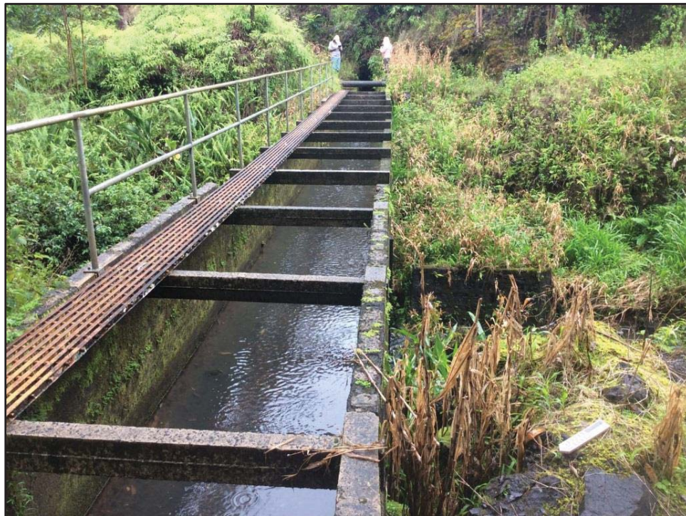
Figure 58. General view of a metal walkway above a flume crossing Waiohue Stream, view to southeast
