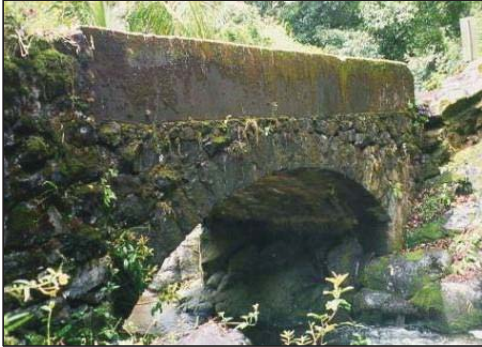
Figure 40. Hāhālawe Bridge, a characteristic masonry arch style bridge (Wilson Okamoto & Associates 2001)
