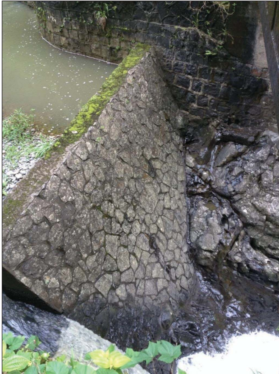
Figure 53. General view of the West Wailuanui diversion dam showing basalt and mortar masonry, view to west
