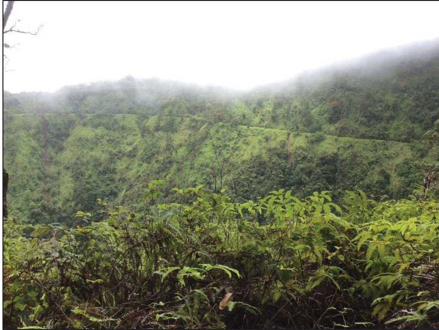
Figure 49. General view of the ditch trail in the vicinity of the Banana sluice gate showing the steep terrain above and below the trail as well as the extend of vegetation cover, view to southeast
