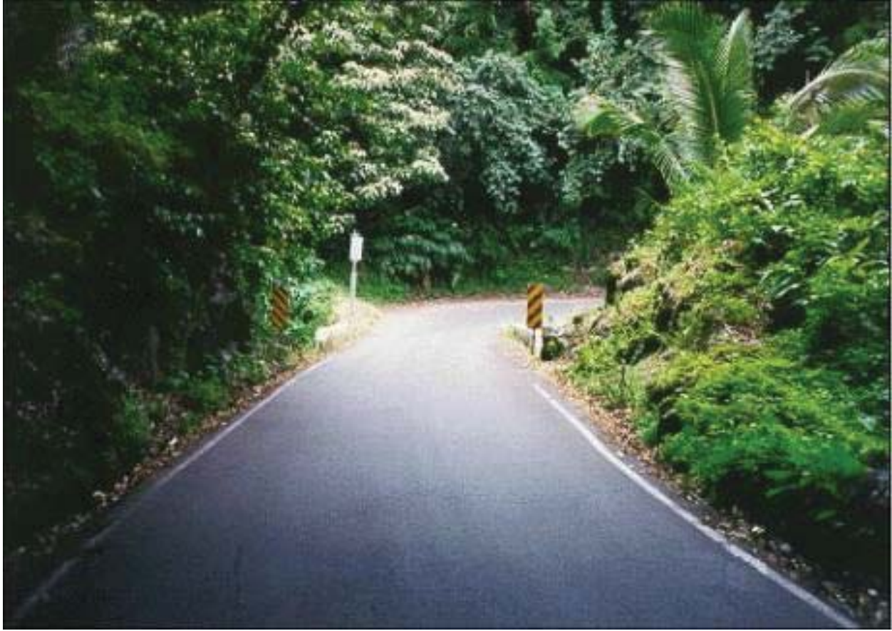
Figure 42. Hāna Belt Road near Waiele Bridge, illustrating the narrow roadway tightly encroached upon by bedrock ridges and jungle vegetation (Wilson Okamoto & Associates 2001)
