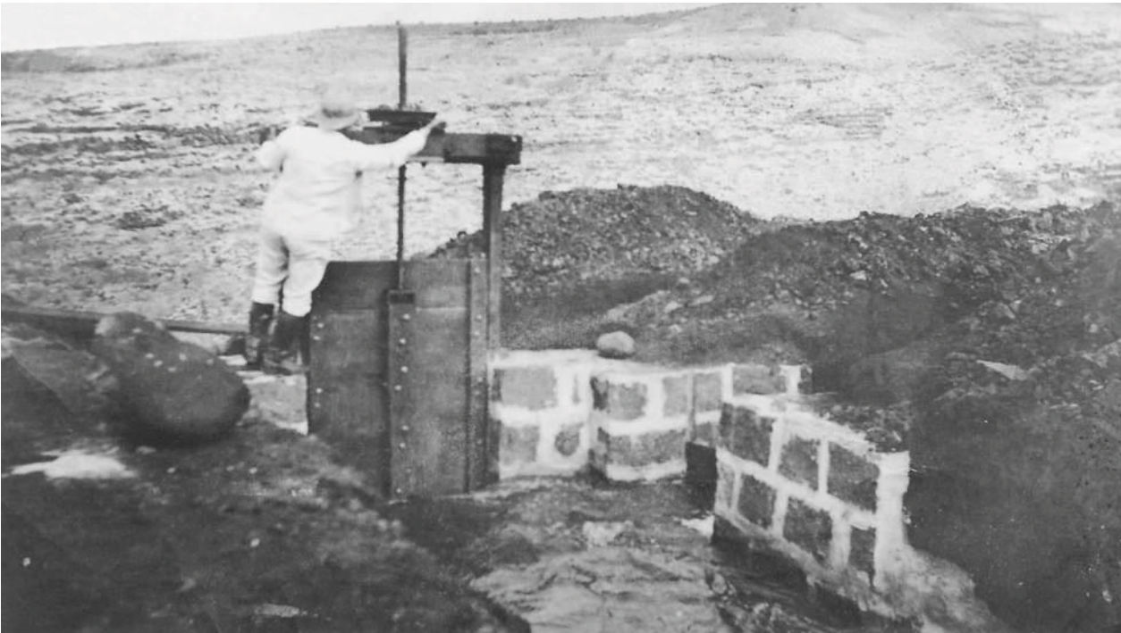
Figure 4: Kekaha Ditch, Kaua'i (possibly above the Mana Plain) ca. 1907. The gate in the photo is the inlet for a siphon. (Source: Private collection of Chris Faye, Kekaha, Kauai)
