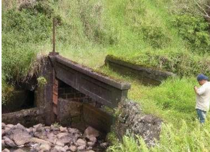
Figure 6: Bridge at Banana Intake stream diversion carries an access trail over the stream. (Source: MAI, 2018)
