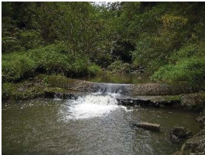
Figure 15: Wailuanui West Stream diversion. View facing SW. (Source: MAI, 2018.)
