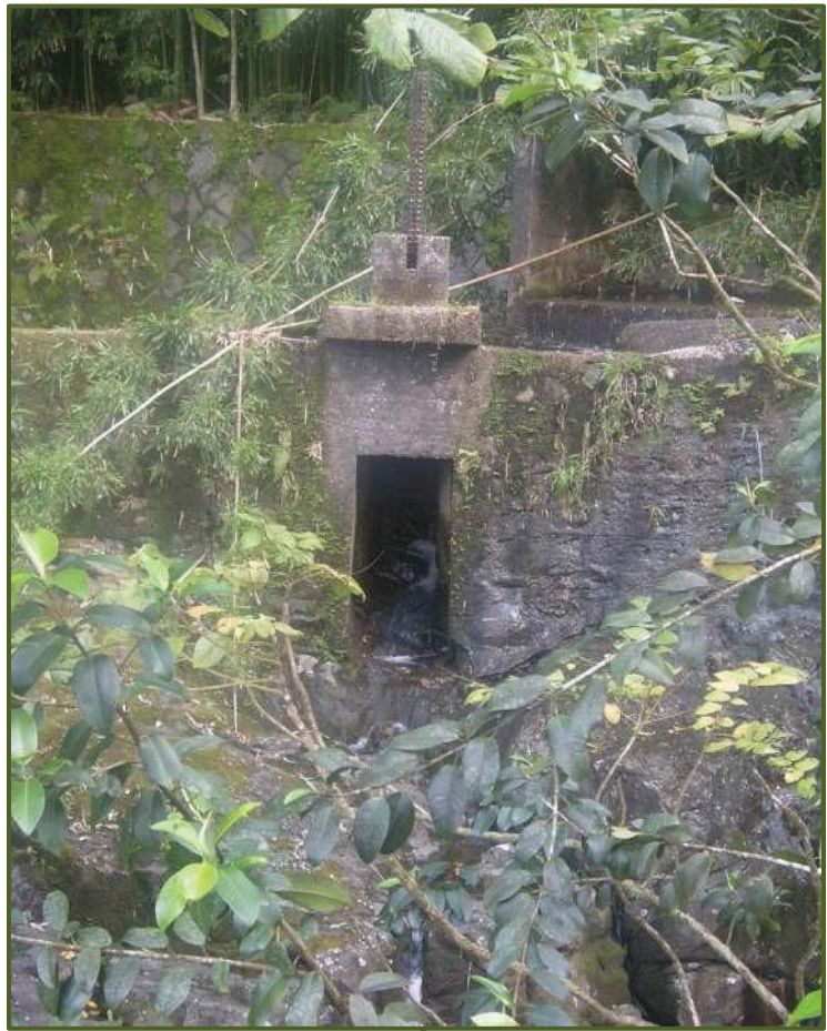
Ratchet sluice gate throw-out at Kaaiea stream diversion. View facing S
