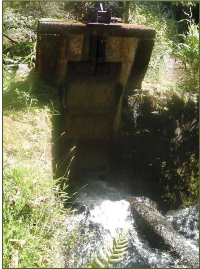
Ratchet sluice gate throw-out at intake of Hoolawa Nui stream diversion. View facing S.
