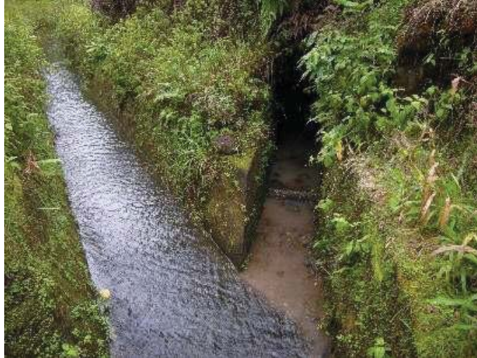
Figure 8: Koolau Ditch near Waiohue Stream diversion. View Facing S. (Source: MAI, 2018)
