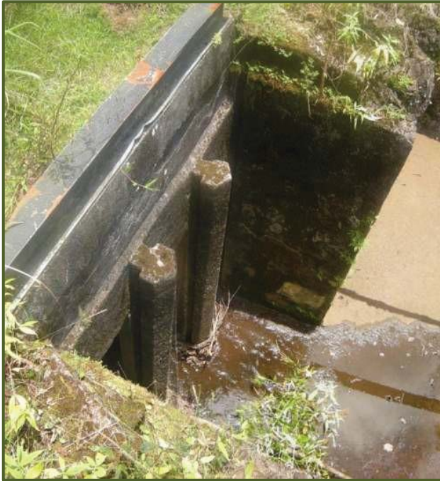
Board adjusted throw-out sluice gate at Piinaau throw-out. View facing NE.
