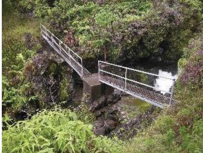
Figure 14: Walkway above Makapipi Stream diversion. View facing S. (Source: MAI, 2018.)
