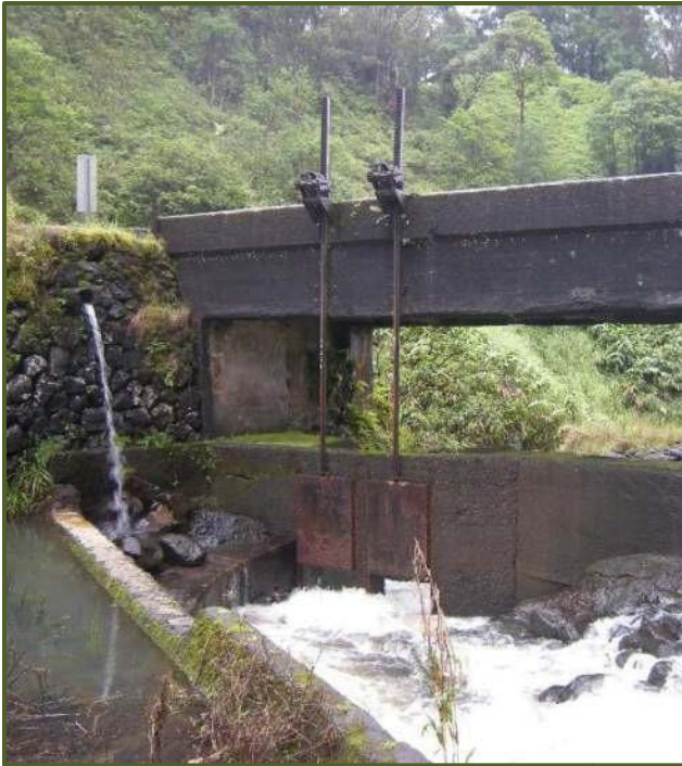
Geared sluice gate at intake at Ko Piliula stream diversion DAM. View facing N.
