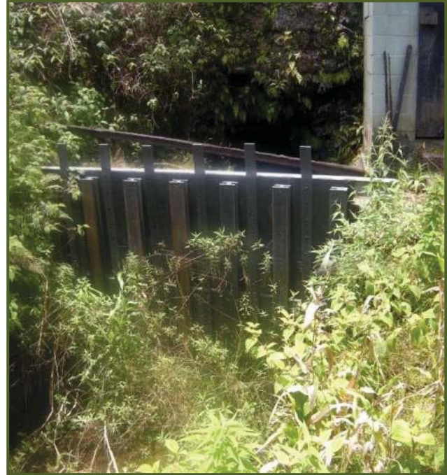
Ratchet sluice gate throw-out at intake of Hoolawa Nui stream diversion. View facing S.
