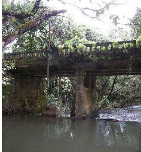
Figure 14: Geared sluice gate at Hoolawa Haiku stream diversion dam. Eligible for the Hawaii Register as a contributing feature to a potential district. Integrity partially retained. View facing NW. (Source: MAI, 2018)
