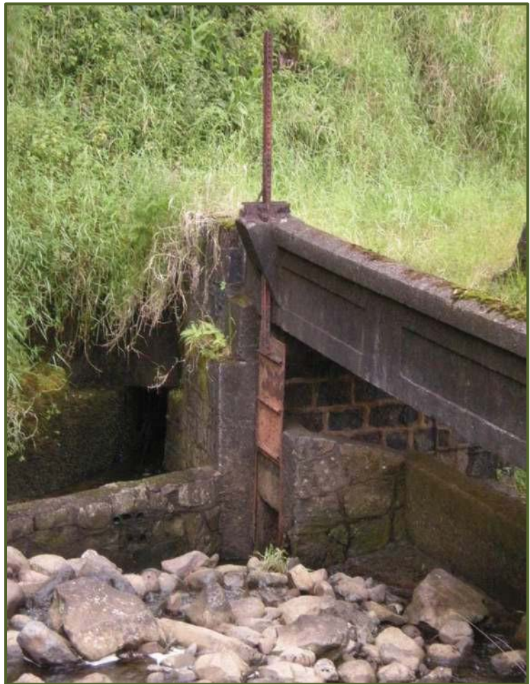
Ratchet sluice gate at Banana Intake stream diversion dam. View facing NW.
