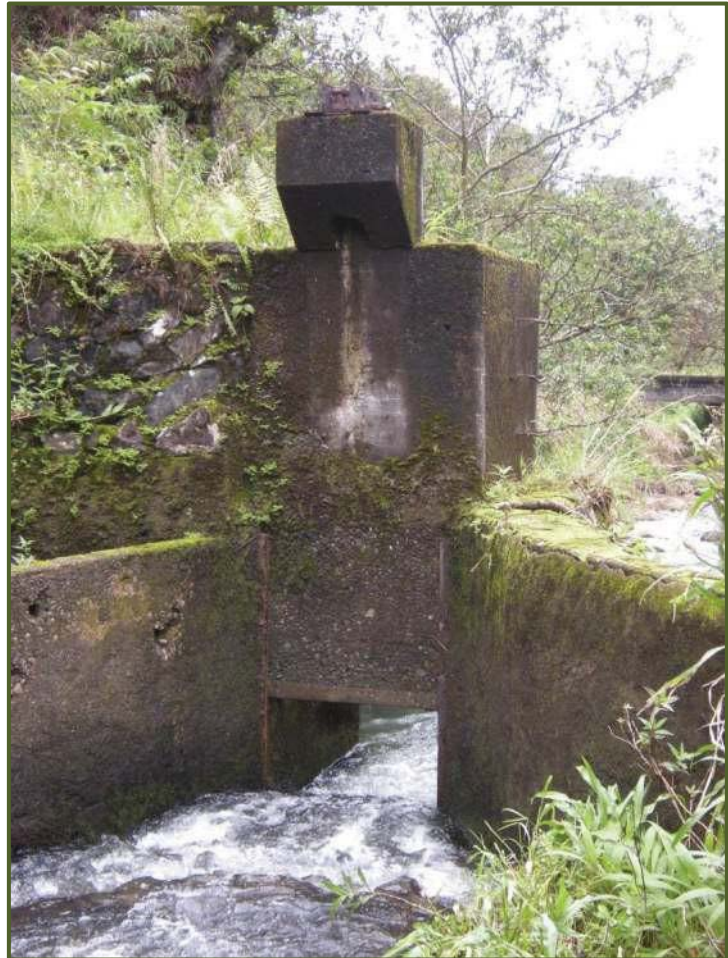
Removed sluice gate (ratchet) at Wailua Nui East stream diversion dam. View facing NE.
