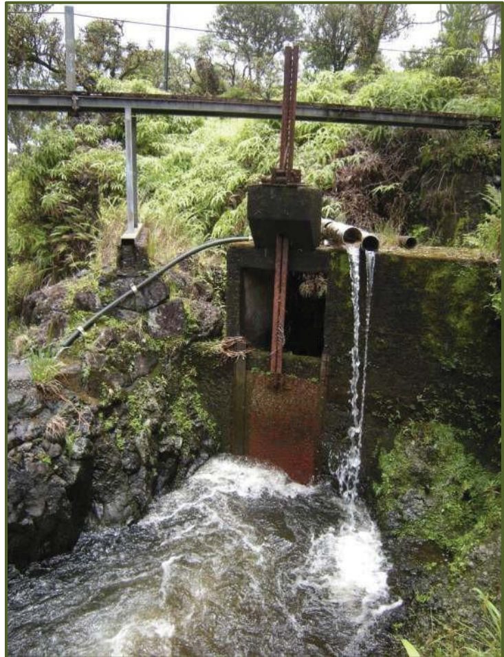
Ratchet sluice gate at Hanawi stream diversion dam. View facing SE.
