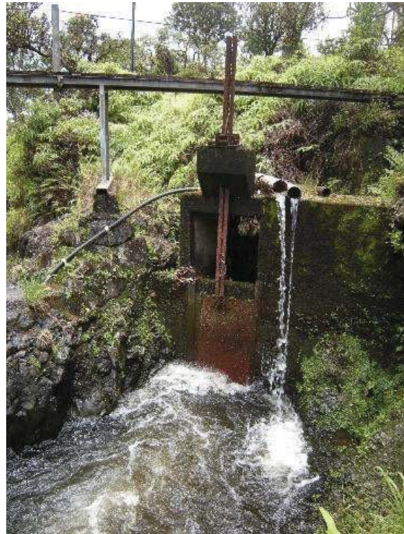
Figure 2: Ratchet sluice gate at Hanawi stream diversion dam. Eligible for the Hawaii Register as a contributing feature to a potential district. Integrity largely retained. View facing NE. (Source: MAI, 2018)
