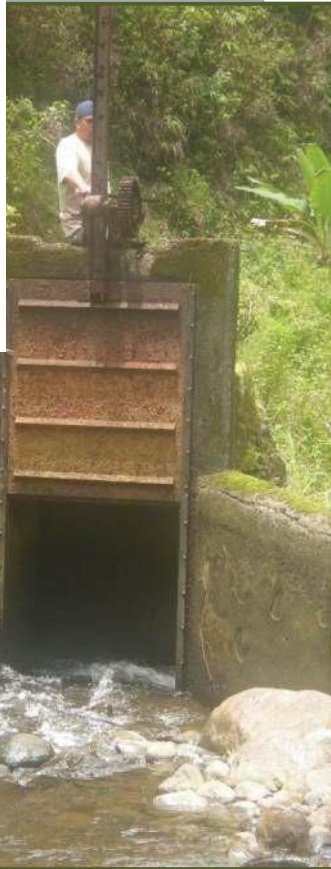
Geared sluice gate at Honomanu stream diversion dam. View facing N.
