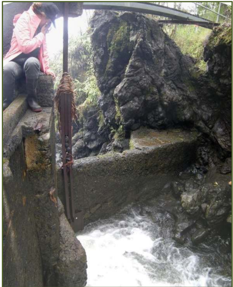
Ratchet sluice gate at Makapipi stream diversion dam. View facing NE. Source: MAI, 2018
