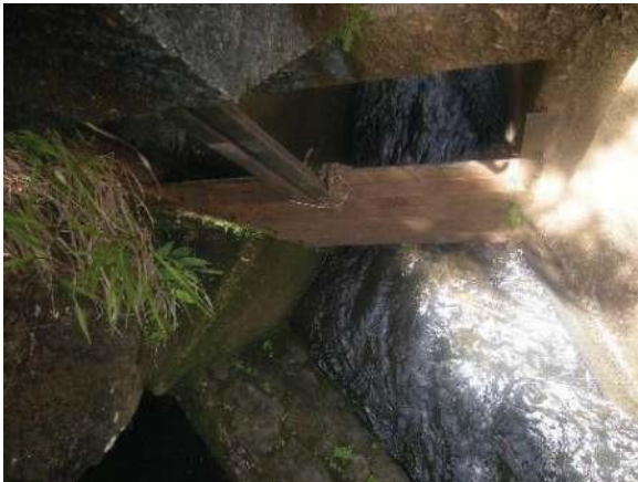
Figure 29: Ratchet sluice gate at Wai Ka Moi stream diversion dam. Eligible for the Hawaii Register as a contributing feature to a potential district. Integrity largely retained. View facing NW. (Source: MAI, 2018)
