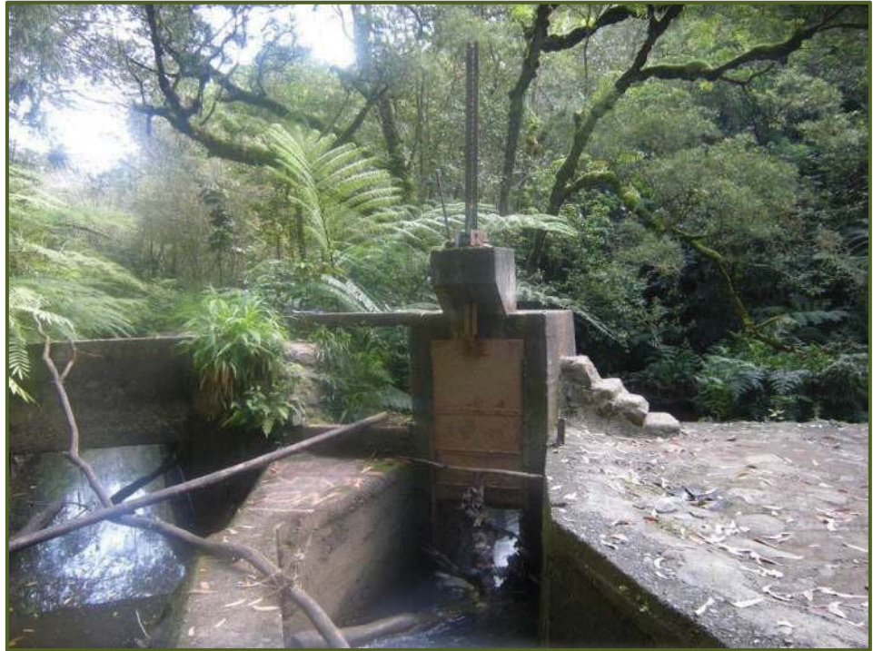
Ratchet sluice gate at Hoolawa Lii Lii stream diversion dam. View facing NE.
