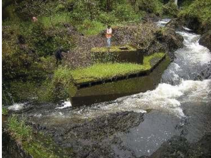
Figure 10: Intake at Hanawi Stream diversion. View Facing S. (Source: MAI, 2018)
