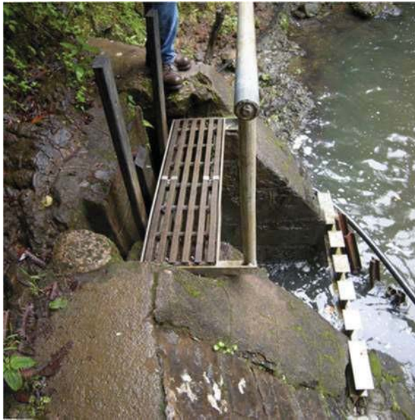
Figure 32: Board adjusted sluice gate with plastic boards installed. Boards are in the closed position, preventing water from passing through the gate. At about 2'-6" wide, this gate is typical width for board adjusted gates seen at EMI during the field survey. This board adjusted gate is located at EMI stream diversion at Waiohue, which is ordered to be a "Fully Restored" stream by CWRM. View facing SE. (Source: MAI, 2018.)
