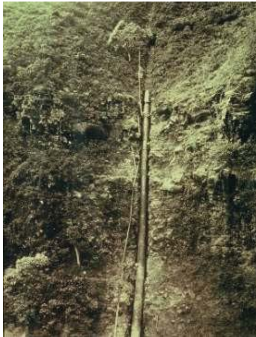
Figure 11: Maliko siphon, unknown date. (Source: EMI archives)
