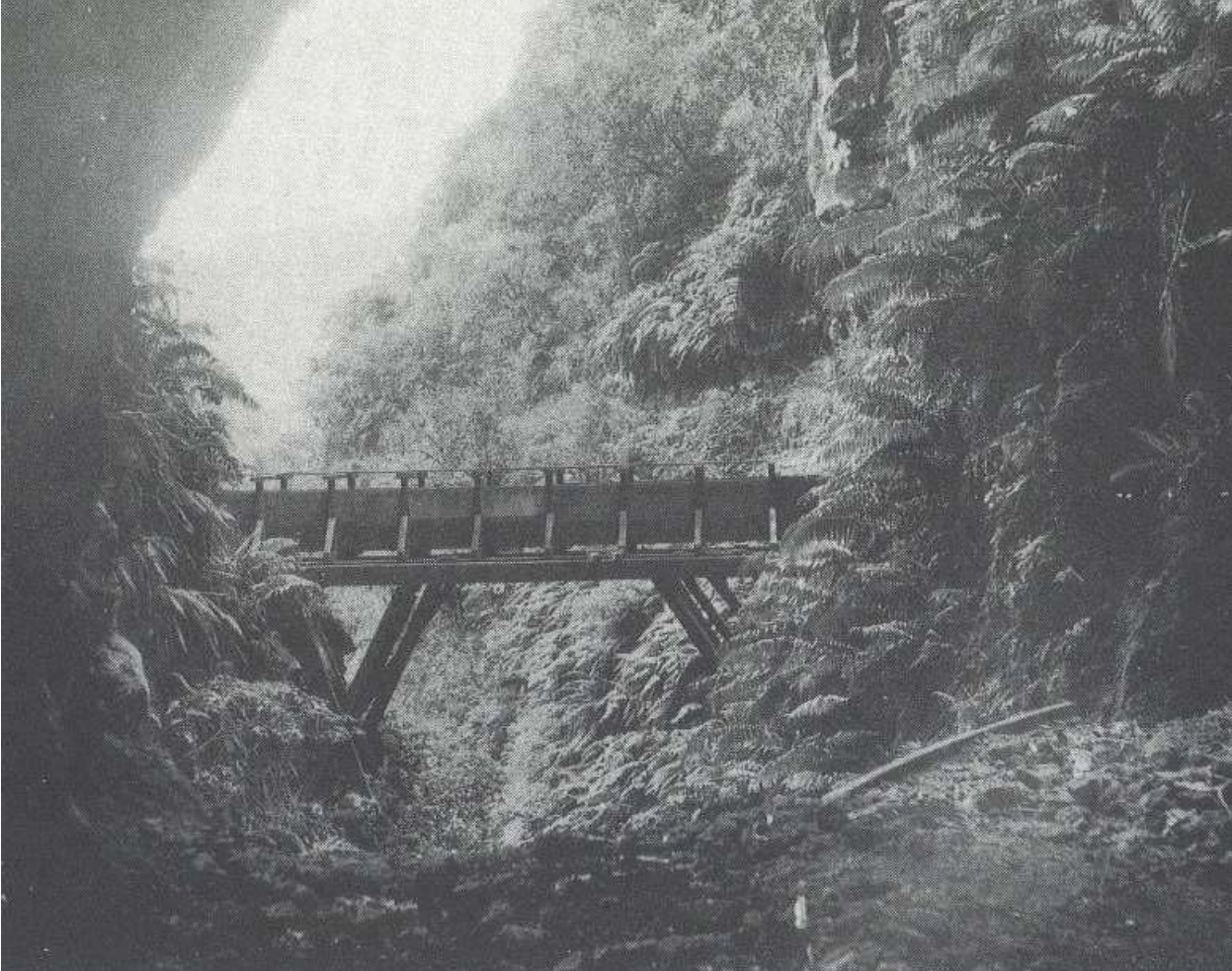
Figure 5: A wooden flume in West Maui. Date unknown. (Source: Wilcox, Sugar Water .)
