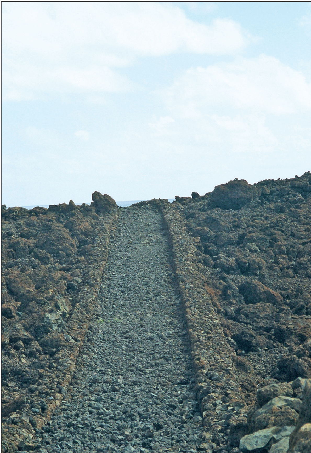
Figure 28 Section of Hoapili trail (c. 1824-1834) built under Governor Hoapili as a horse and cart route over the lands of Kula, Honua'ula, Kahikinui and Kaupo. In many places the trail overlaid the older Ke Ala Loa from Pi'ilani's time. 2002.
