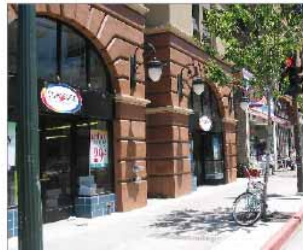
High glass doors with metal frames in Mixed-Use building
