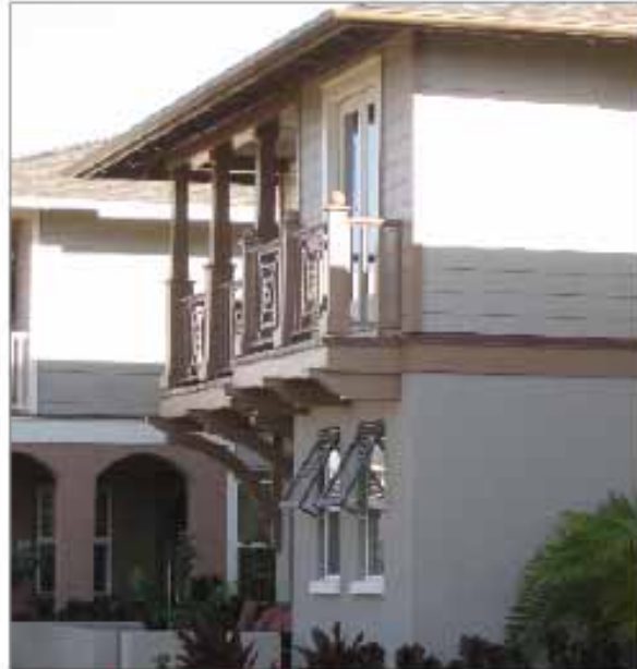
Decorative Braces and Window Shades
