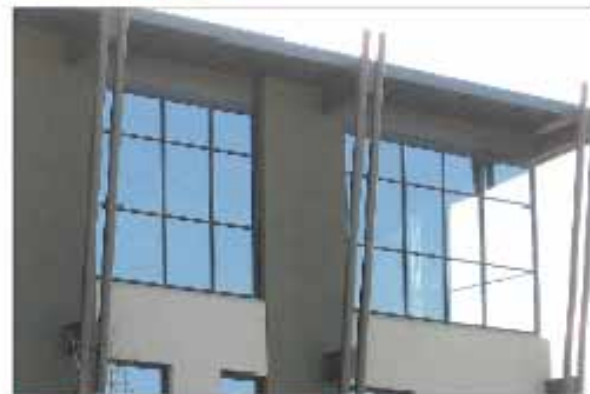
High glass windows for lighting in Office building
