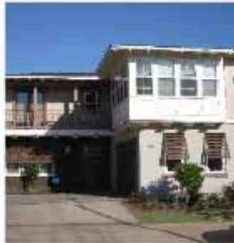
Variety of wall materials, textures and treatments used modernly
