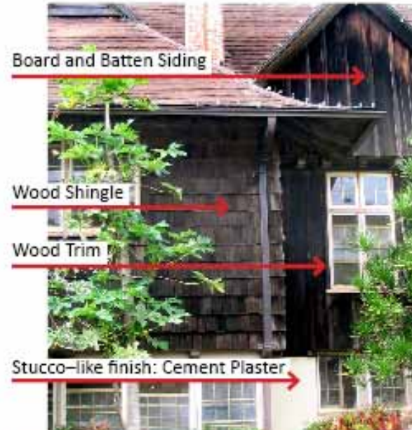
Variety of wall materials, textures and treatments used traditionally
