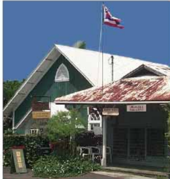
Single-Pitched Hipped and Gabled Roof in Honolulu
