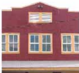
Traditional use of framing and wall material
